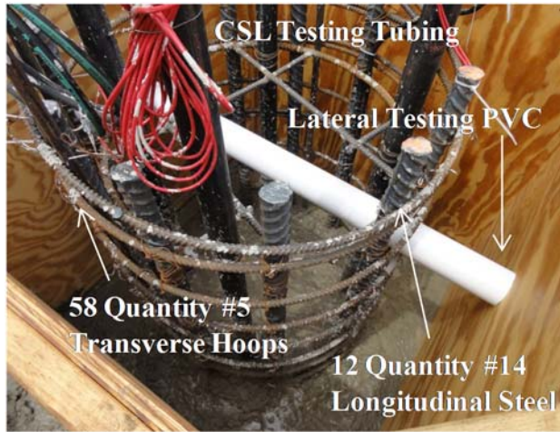
Figure 5.22. Photographs of the Test Shaft SS-E4 (a) rebar cage and pipe for lateral load testing, and (b) finished construction.
