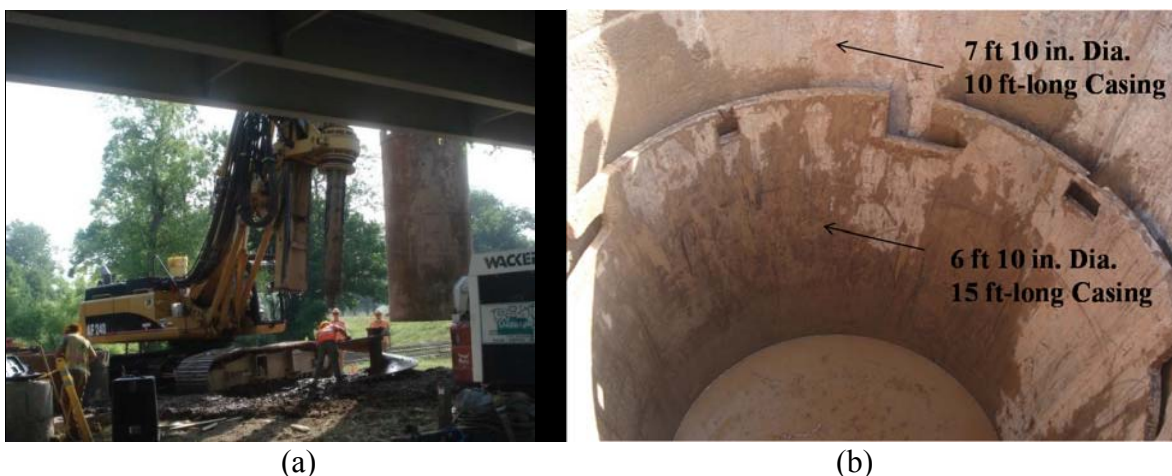
Figure 5.16. Photographs of Test Shaft SS-C6 (a) during the 15 foot length casing installation, and (b) after completed casing installation.
