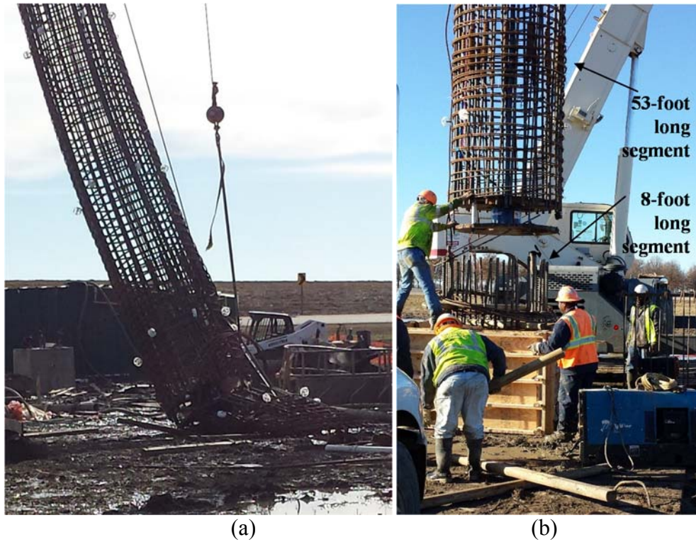
Figure 6.29. Photograph of test shaft T-C6 during the (a) second un-successful pick, and (b) second re-assembly process.
