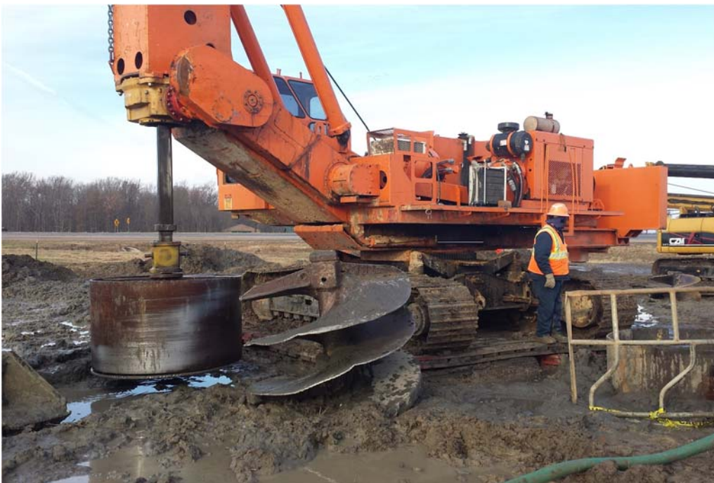
Figure 6.20. Photograph of the imported Watson AGBO G150 drill rig.
