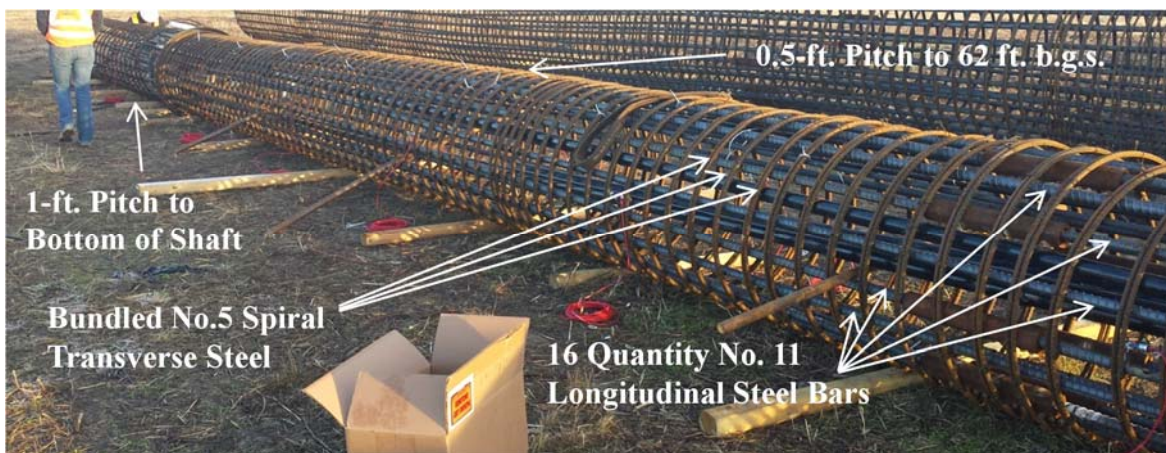
Figure 6.3. Photograph of a four-foot diameter shaft reinforcement cage from the side view.
