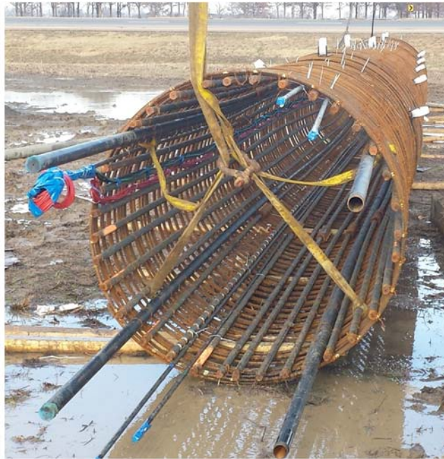
Figure 6.27. Schematic of (a) top-down view of test shaft T-C6, and (b) photograph of instrumented assembly.
