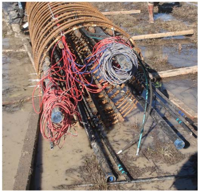
Figure 6.39. Schematic of (a) top-down view of test shaft T-N4, and (b) photograph of instrumented assembly.
